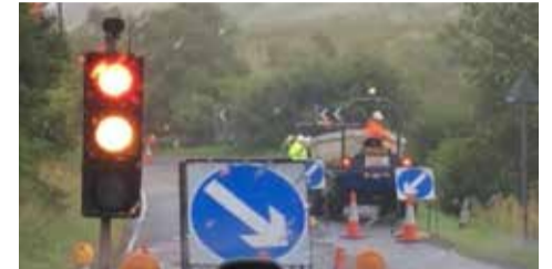
The HS2 ground work investigations begin
